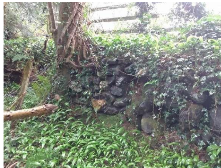
Plate 4 Stone boundary wall, facing northwest
